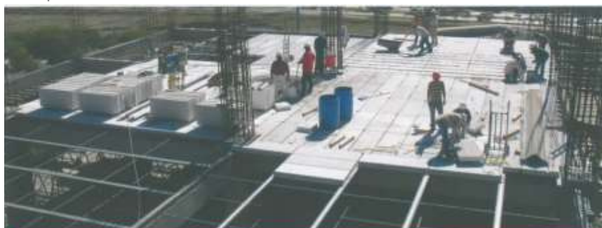
Fig. 5: Slab Panels supported by steel elements
