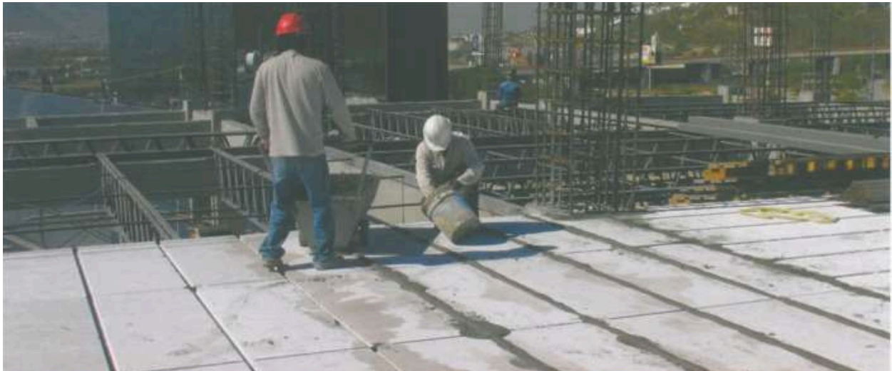
Fig. 18: Filling Longitudinal joints with cement-sand mortar
