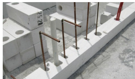
Fig. 25: Water supply pipes.
