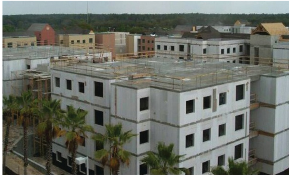
Fig.28:Builtusing Hebel® Masonry Components.
