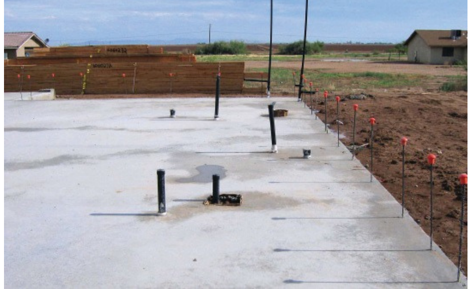
Fig. 6: Check foundation (pipes, drains, reinforcement, etc).
