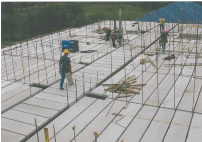
Fig. 15: Five story hotel built with AAC (Floor Panel)
