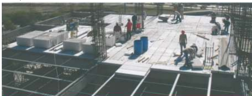
Fig. 5: Slab Panels supported by steel elements
