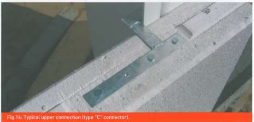
Fig.14: Typical upper connection [type "C" connector].
