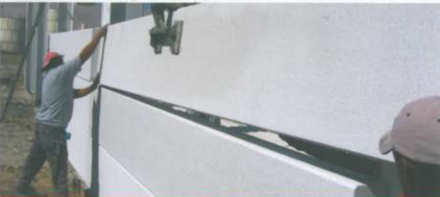
Fig.10: Sliding second panel.
