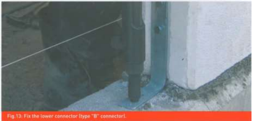
Fig.13: Fix the lower connector [type "B" connector].
