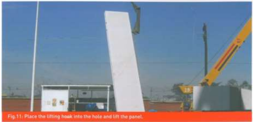
Fig.11: Place the lifting hook into the hole and lift the panel.
