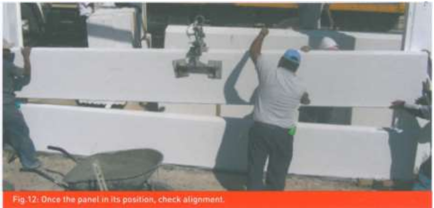
Fig.12: Once the panel in its position, check alignment.
